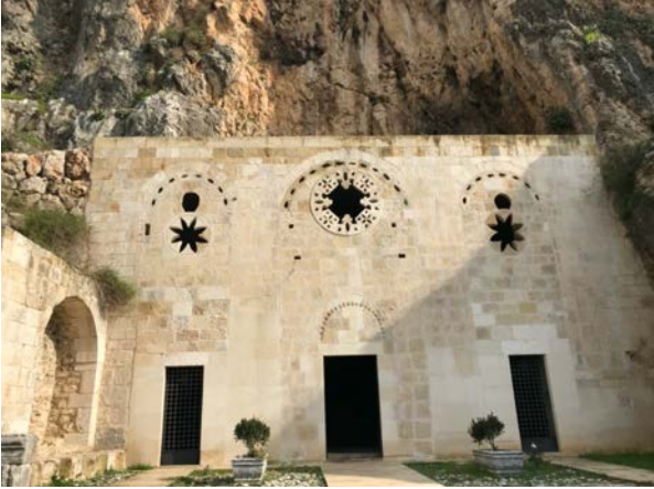
Saint Pierre's Church, Antakya
